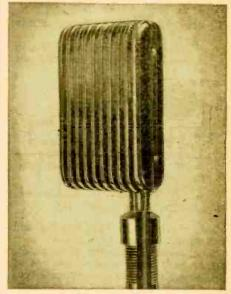
Fig. 3-A tube transducer type microphone.
