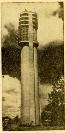
A MICROWAVE TOWER "to bring into the laboratory the facilities of the field" was dedicated by Federal Telecommunications Laboratories last month at Nutley, New Jersey. Rising 300 feet from its base and 358 feet above sea level, it will make possible the carrying on of many experiments right at the best point for a radiator.
