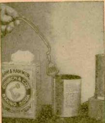
Fig. 10-Baking soda removes the corrosion.
